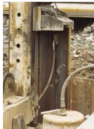
Piling element with mounted high-pressure lance and high-pressure hose
