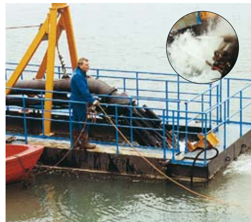
Waterjet system for pushing through clay layers in gravel pits
