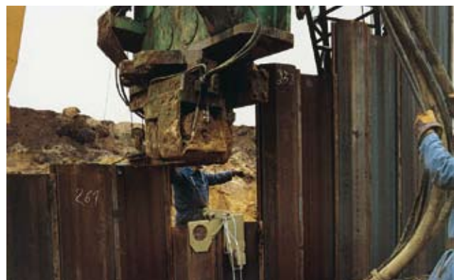
Pile elements at the Hamm-Dattel-Canal, driven with waterjet assistance
