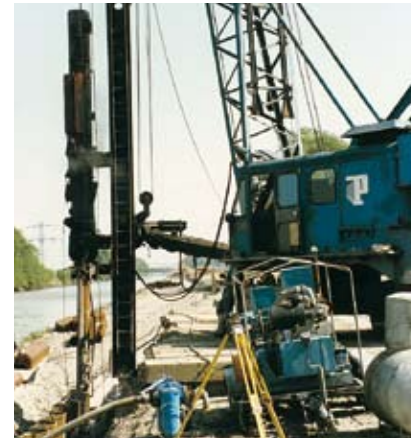
Diesel pile driver with a WOMA high-pressure waterjet system
