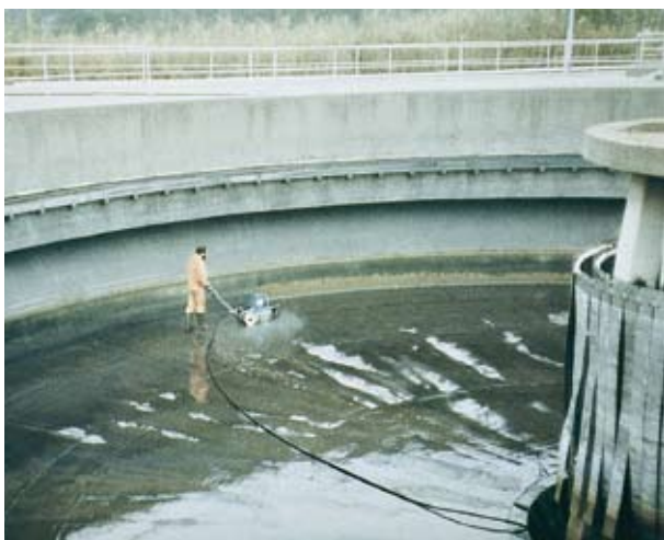
Cleaning of settling basins
