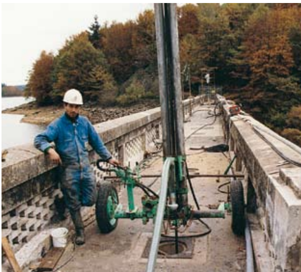
Pipe cleaning by an TubeMaster®-System and vertical traverse unit
