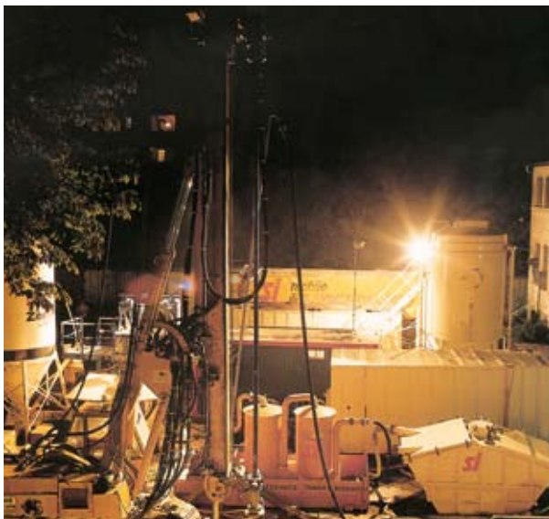
Decontamination of phenol-contaminated soil with WOMA's high-pressure technique
