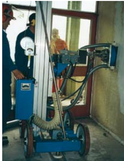
Emission-free removal of PCB-contaminated plasters
