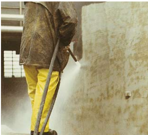
Chromium oxide removal from heat barriers of a nuclear power plant
