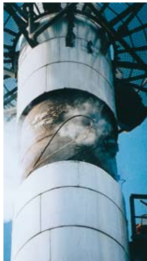
Demolition of double-walled steel structures
