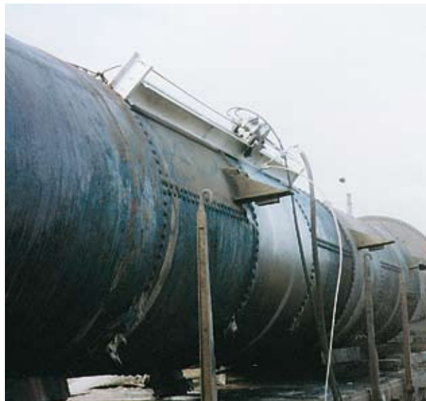
Cutting openings in large storage vessels
