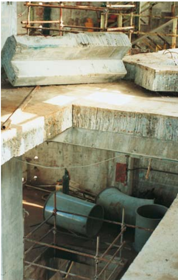
Partial demolition of heavily reinforced concrete ceilings
