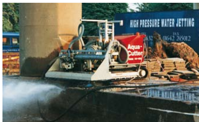
Heavy hydrodemolition of concrete with specially developed high-pressure robots
