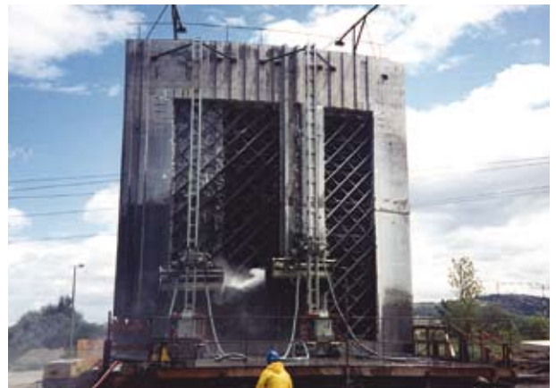
Heavy concrete hydrodemolition
