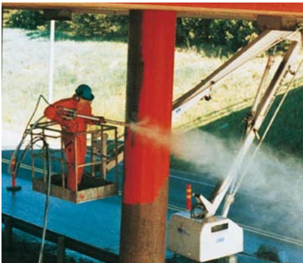
Decoating of reinforced concrete with hand-held high-pressure water jet guns
