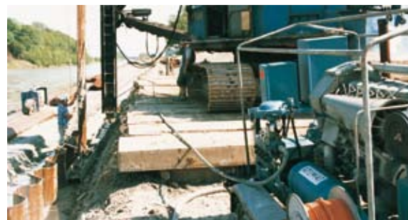
High-pressure water jet supported sheet pile driving
