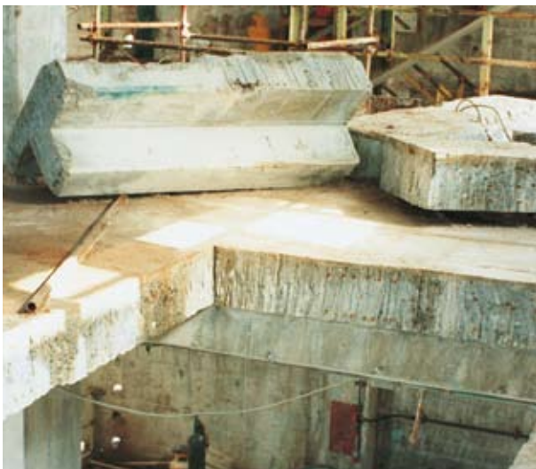
Vibration-free cutting of reinforced concrete floors by abrasive high-pressure water jets
