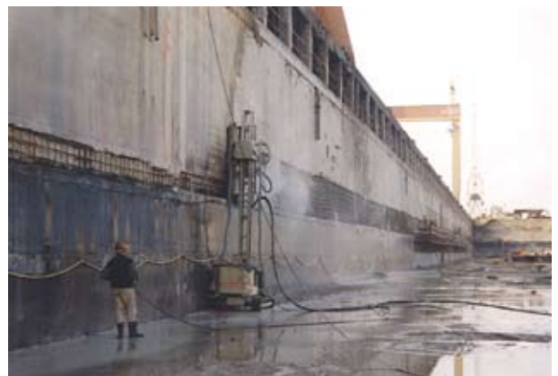
Concrete hydrodemolition in drydocks
