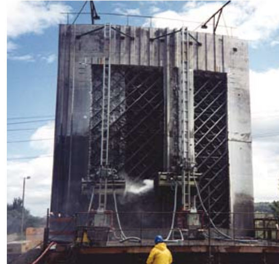
Heavy concrete hydrodemolition
